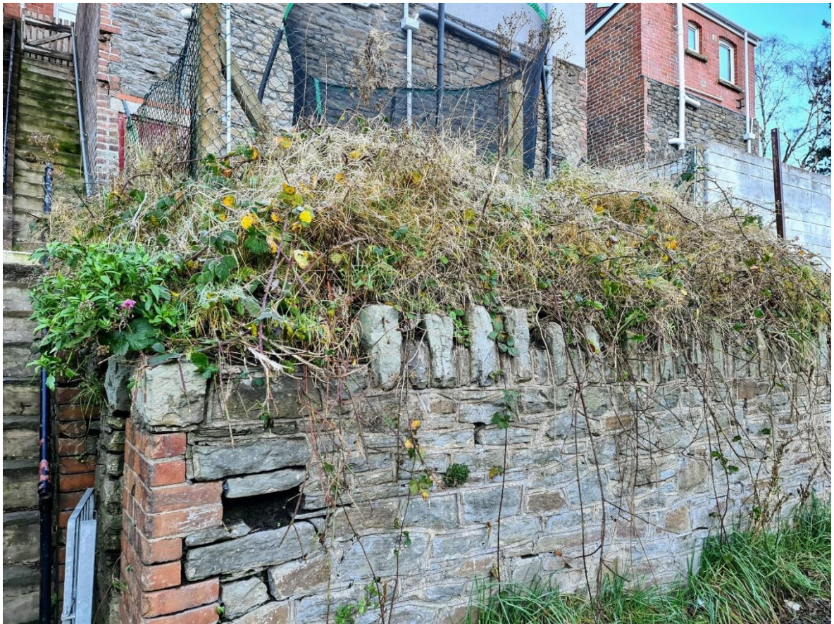
Examples of Rear Retaining Walls
